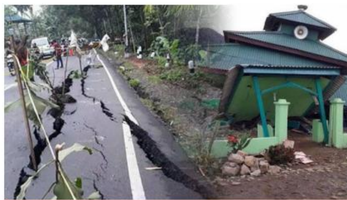
Figure 3. Building Damage Due to Foundation Failure During the Pandeglang Earthquake, 24 February 2024
