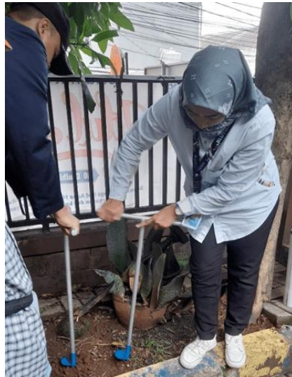
Figure 10. Biopore installation practice
