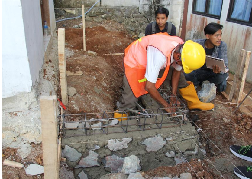
Figure 5. Training connection and rebaring between foundation and sloof
