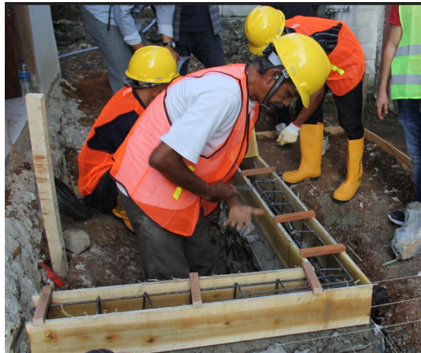
Figure 6. Training installation formwork of sloof
