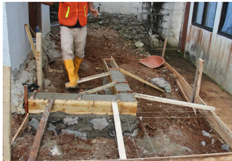
Figure 7. The final result of field training installation connection foundation and sloof
