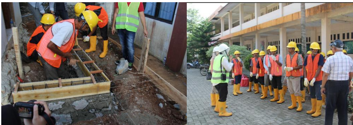
Figure 6. Construction methods: (a) proper installation of tie beam formwork; (b) instruction on the use of personal protective equipment (PPE).
