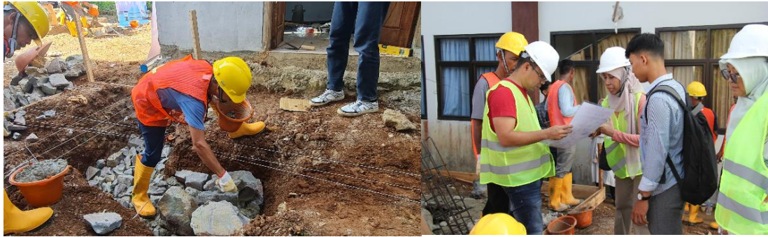
Figure 7. Foundation implementation: (a) field practice of shallow foundation construction following correct procedures; (b) reflection and discussion on construction sequence using Work Breakdown Structure (WBS).
