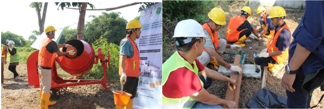
Figure 5. Substructure practice: (a) concrete mixing with a 1:2:3 ratio; (b) reinforcement bending with 40D anchorage length.
