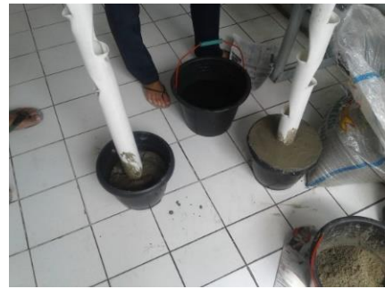
Figure 10. Pipe support casting
