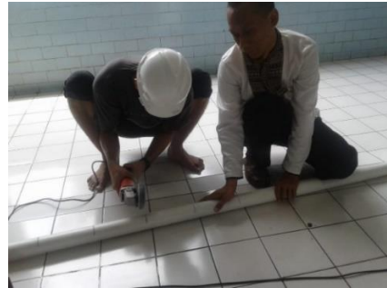
Figure 7. Pipe cutting according to the mark
