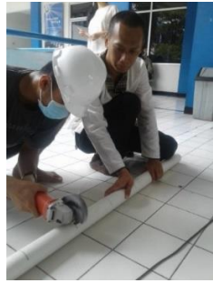
Figure 7. Pipe cutting according to the mark
