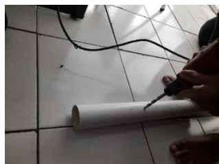
Figure 12. Making ventilation holes for water at the bottom of the pipe
