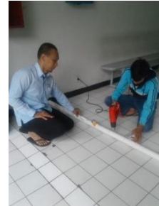
Figure 8. Heating the cut part using an acrylic heater
