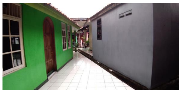
Figure 5. Left Facade of Al Hasanah Mosque
