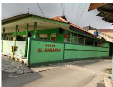
Figure 4. Right Facade of Al Hasanah Mosque
