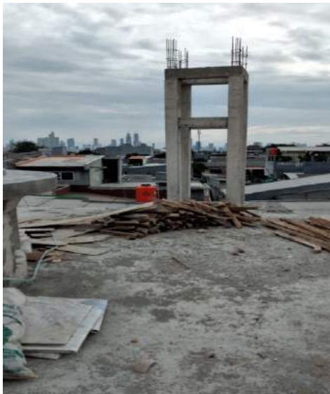
Picture 28. Reinforced concrete structure Tower of flat roof floor.
