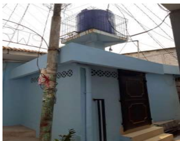
Picture 3. West side facade of Mushollah Al Ikhlas
