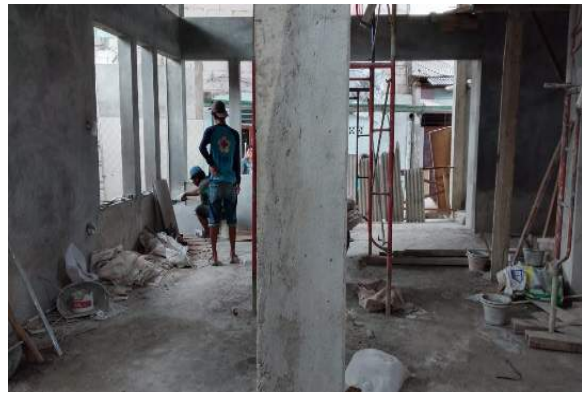
Picture 24. Prayer Room Area on the 1st floor after renovation
