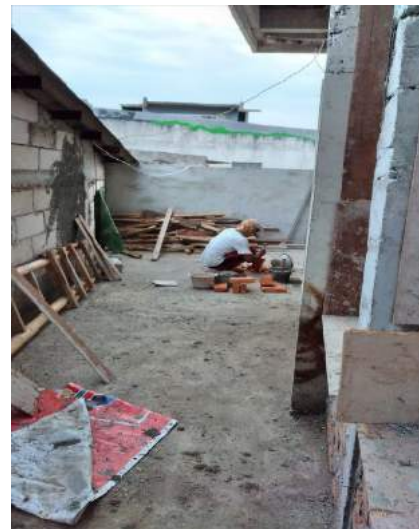
Picture 27. The 2nd floor pavilion which is on the south side
