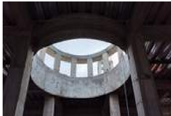
Picture 26. Dome support structure
