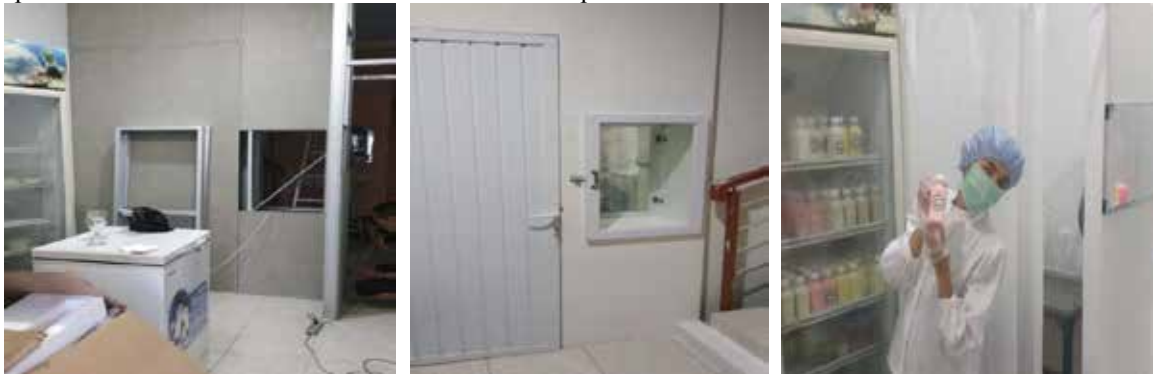
Picture 2. Rumah yogurt's kitchen renovations
