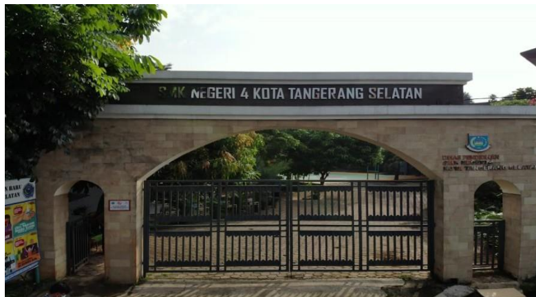
Figure 2. Gate's School of SMK Negeri 4 Tangerang Selatan
