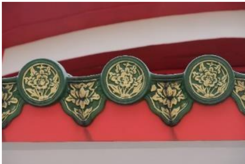
Fig. 10. Hua tou ban wa, 華頭匾瓦, hua bian wa, 花邊瓦, curved rooftile.
