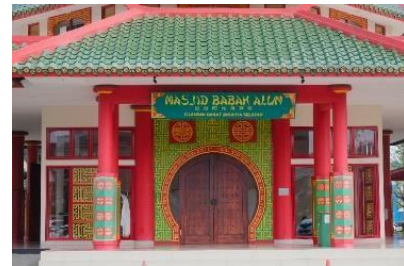
Fig. 13. The red color is widely applied to the column and connection structures.
