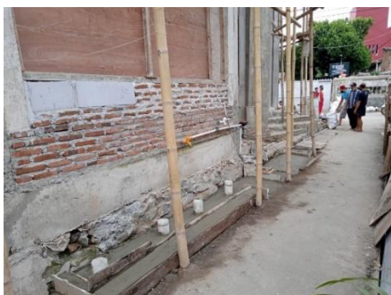
Figure 4 Women's Wudhu Place which is still under construction
