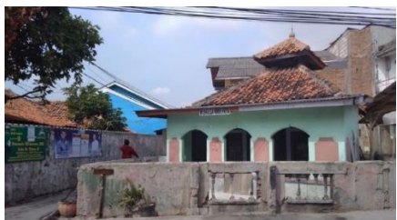
Figure 1 The condition of the Nurul Fata Mushalla building before the renovation
