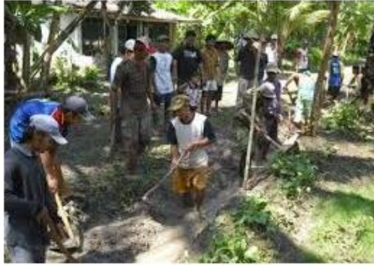
drainage drain repair
